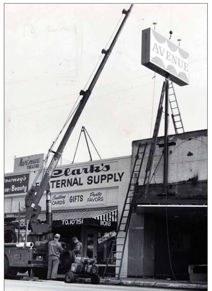
The Avenue Theatre was built in 1922 and has undergone several renovations but would not meet today's seismic requirements, city officials say. Supporters of the theater's renovation disagree. Photo courtesy Downey Historical Society
