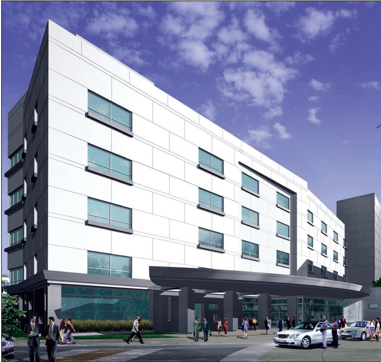
COMING SOON? – Downey Regional Medical Center is attempting to raise $60 million to build its proposed Patient Care Tower, a state-of-the-art medical facility that will offer a ‘homelike’ setting for patients. The hospital’s current facility does not comply with seismic laws set to go into effect this decade.
