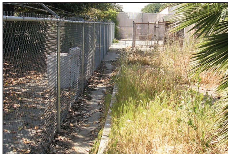
Rose Float officials say an empty strip of grass near their warehouse is home to transients, which break into abandoned warehouses and steal copper wiring. Photo by Eric Pierce
