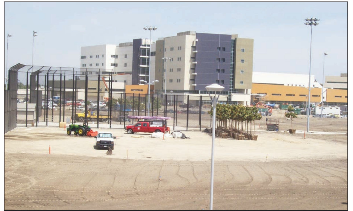
The city is using black chain link fence at the Discovery Sports Complex, which sits between the Columbia Memorial Space Science Learning Center (CMSSLC) and Kaiser Permanente's new medical offices.
