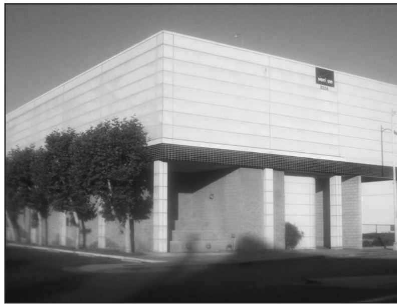
The City Council, with an eye towards revitalizing and reinvigorating the Downtown Downey area, this week authorized the purchase of the vacant Verizon building on 2nd Street. Photo by Brooke Karli
