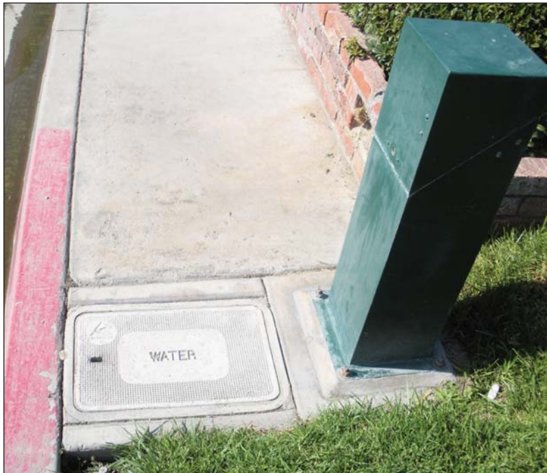
Twenty-five water sampling stations, like the one pictured above, are scattered throughout the city. The city tests each location weekly to satisfy government regulations. Photo by Mary Forney
