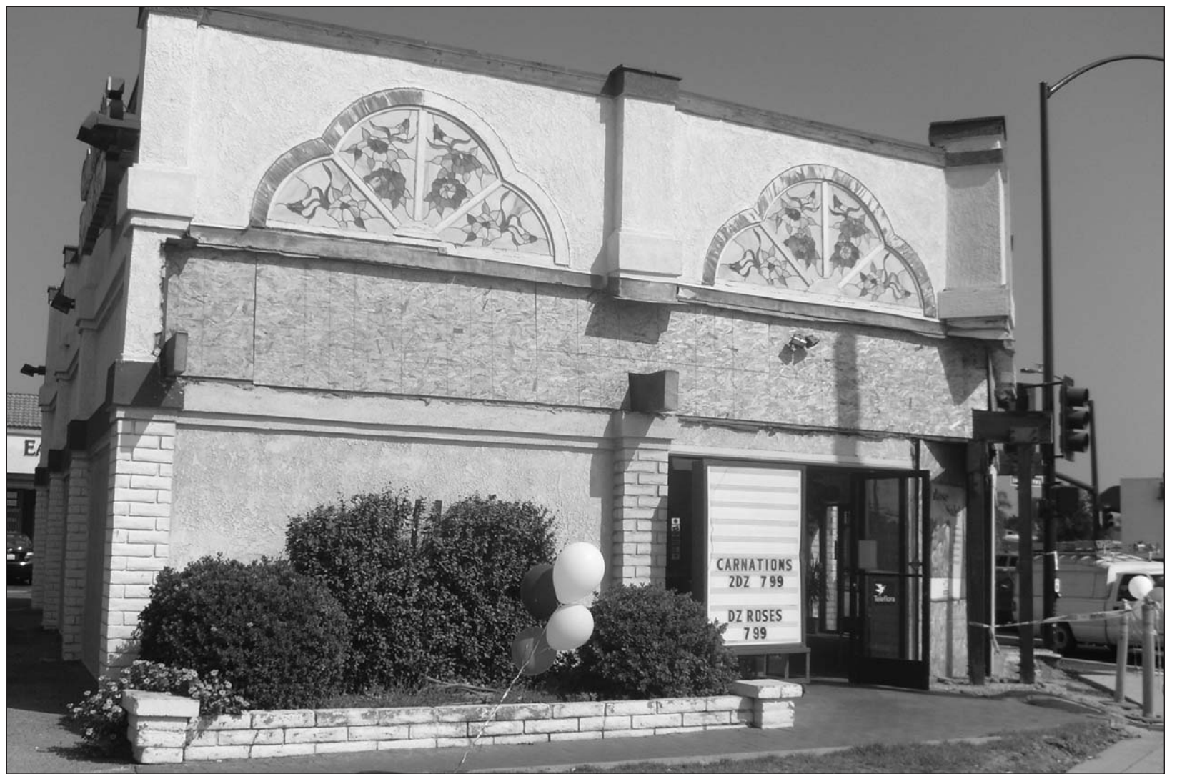
Conroy's Flowers at Lakewood Boulevard and Imperial Highway received a "big ugly scar" as a result of a street-widening project that was supposed to be completed in September. Photo by Mary Forney
