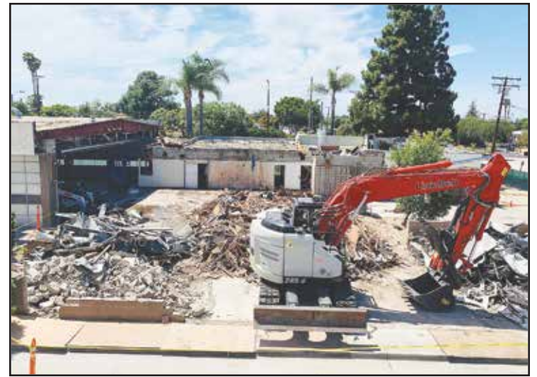
Demolition of Downey Fire Station 1 in 2019.
