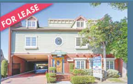
Prime Office Space On Florence
