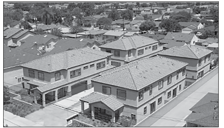
With funding, Cerritos College says it is ready to build affordable housing for over 400 students. The Village is pictured above.
