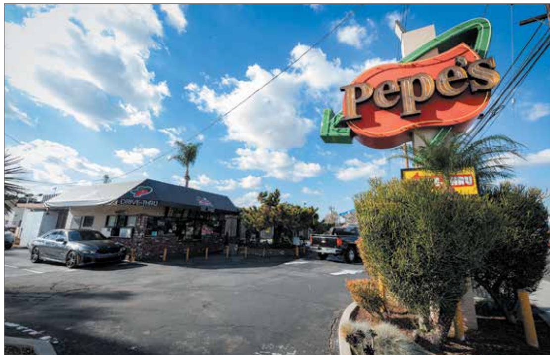
Pepe's Mexican restaurant is expected to close next year although they hope to open at a new location in Downey. Located at 9020 Telegraph Rd., Pepe's has operated since 1974. The corner is slated to be redeveloped into a new Raising Cane's drive-thru restaurant.
