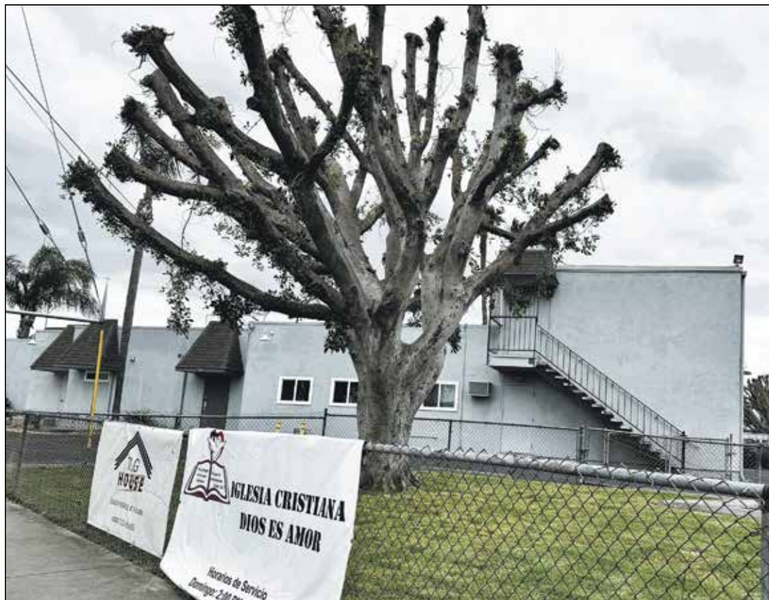
The property at 7360 Foster Bridge Rd. has operated as a church since 1959. The church is moving and there is a proposal to fill the land with condos. Photo by Eric Pierce
